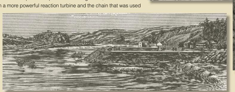
To the left a canal boat is shown leaving the cradle car at the bottom of Inclined Plane 11 West. In the distance an other boat just inside the stone arched entrance waits to across the river by the cable ferry.
